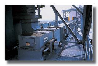
where capacity requirements are fairly high, 200 - 400 TPH and when the material is somewhat fluid. The typical materials conveyed are TSP (fertilizer), raw meal, and finish cement.
